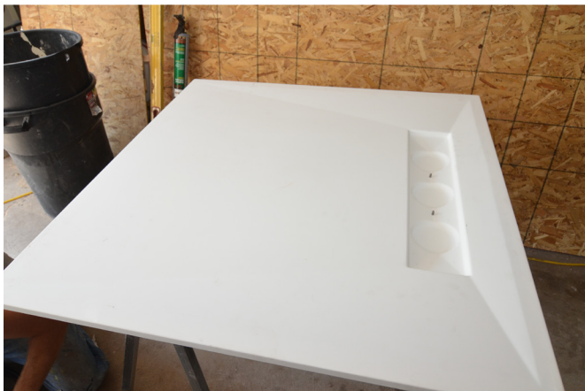
Linear shower foundation showing four gradients and three outlet locations in drain gully.
