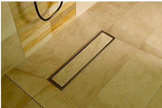
Linear drain—cover filled with tile.
