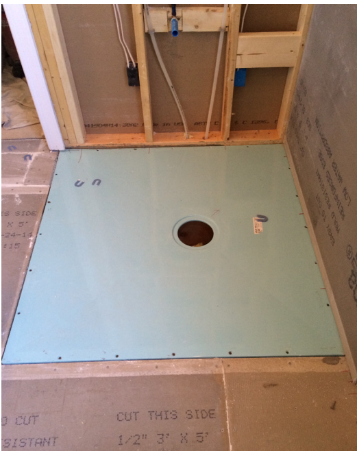
Classic shower foundation installed on joists.
