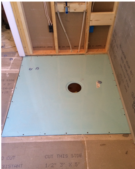
Classic shower foundation installed on joists.
