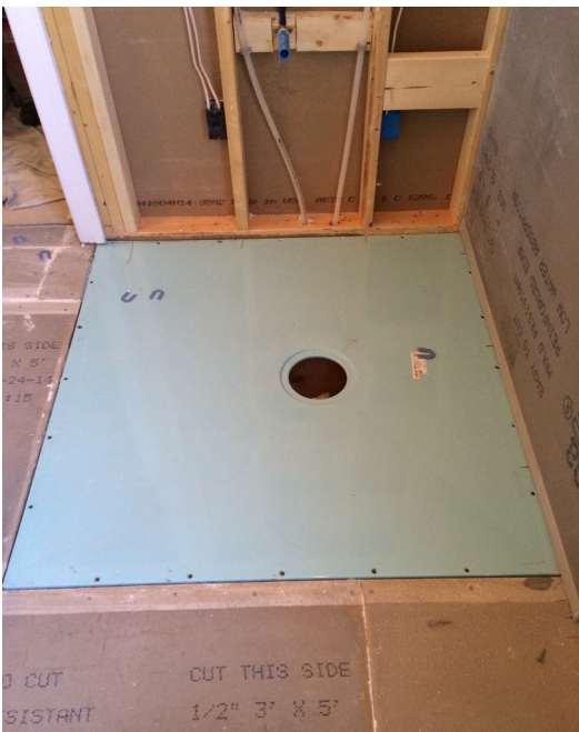
Classic shower foundation installed on joists.
