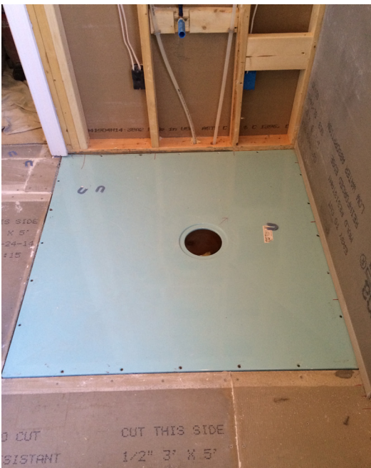
Classic shower foundation installed on joists.
