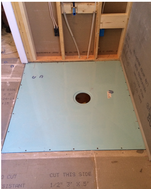
Classic shower foundation installed on joists.
