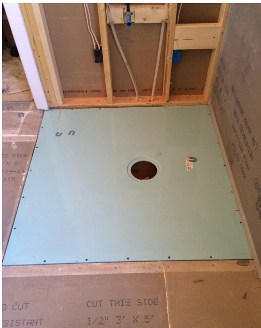
Classic shower foundation installed on joists.
