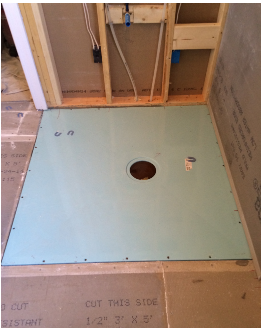
Classic shower foundation installed on joists.
