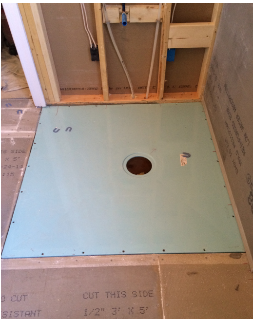
Classic shower foundation installed on joists.
