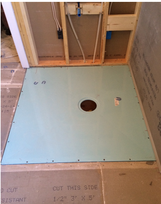
Classic shower base installed on joists.
