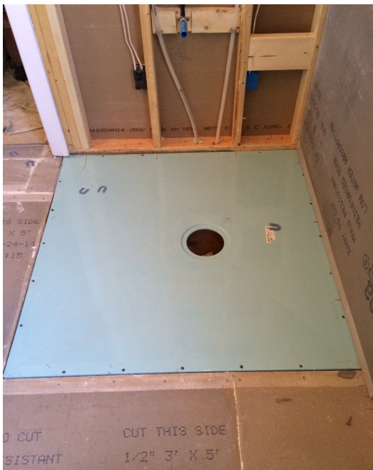
Classic shower base installed on joists.
