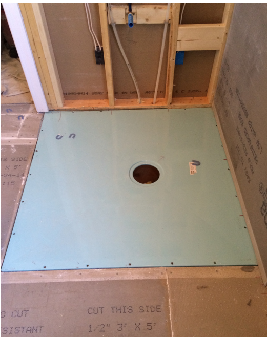
Classic shower base installed on joists.
