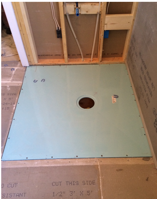
Classic shower base installed on joists.
