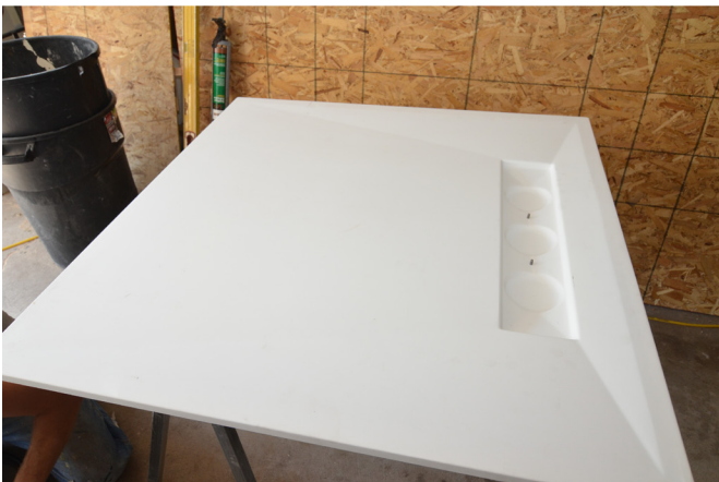
Linear shower base showing four gradients and three outlet locations in drain gully.
