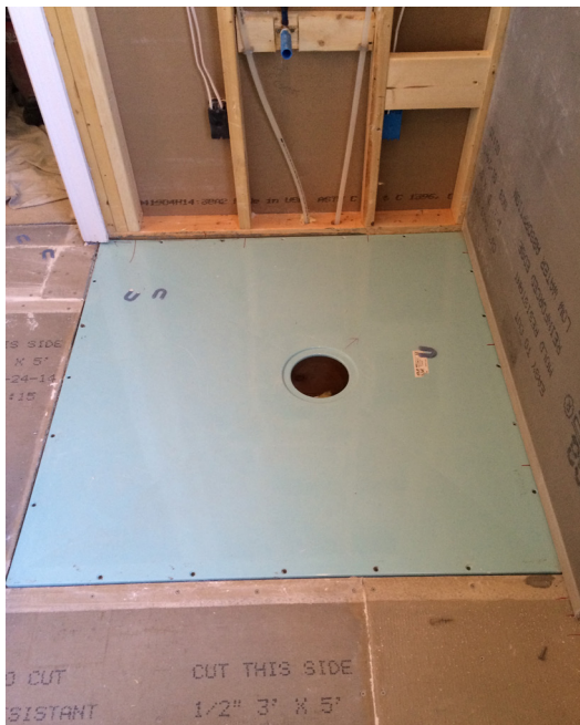
Classic shower base installed on joists.
