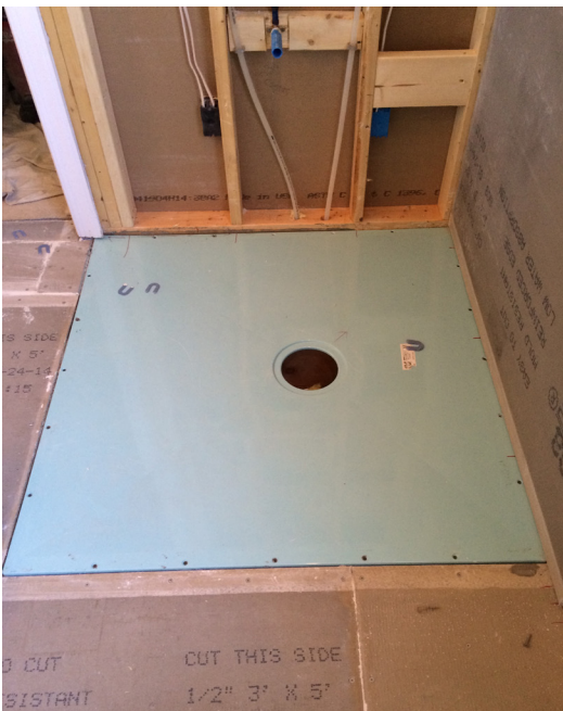
Classic shower base installed on joists.
