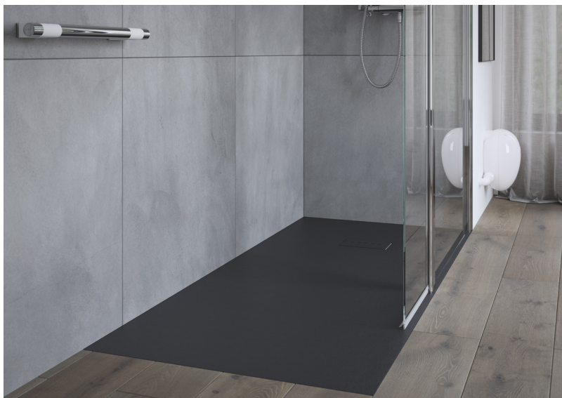
FastDEK installed on finished floor.
